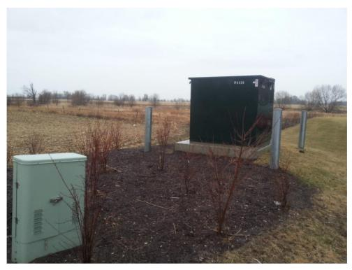
Photograph 11: Pad mounted transformer #2 (located southwest of the grocery store building).
