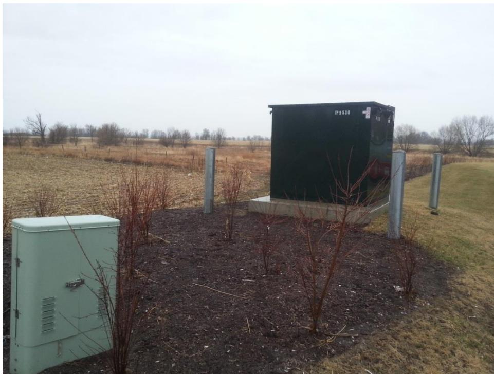
**Photograph 11:** Pad mounted transformer #2 (located southwest of the grocery store building).
