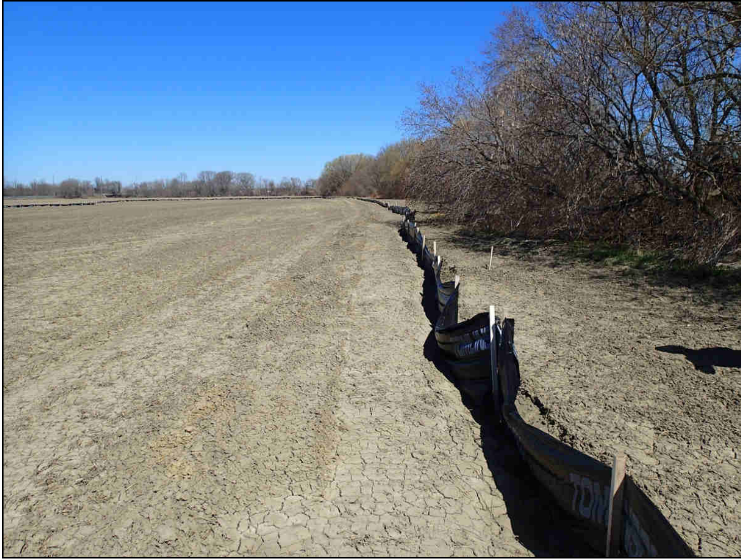
Plate 5: East side of west field looking south.
