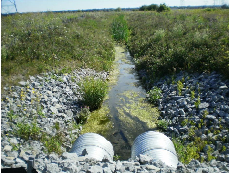
Photo 1 – Realigned portion of the West Tributary downstream of the new high school. View looking east
