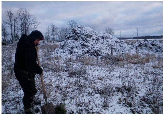
Plate 5: Test pitting; note pile of wood chips as a result of disturbance related to grubbing of wooded areas.
