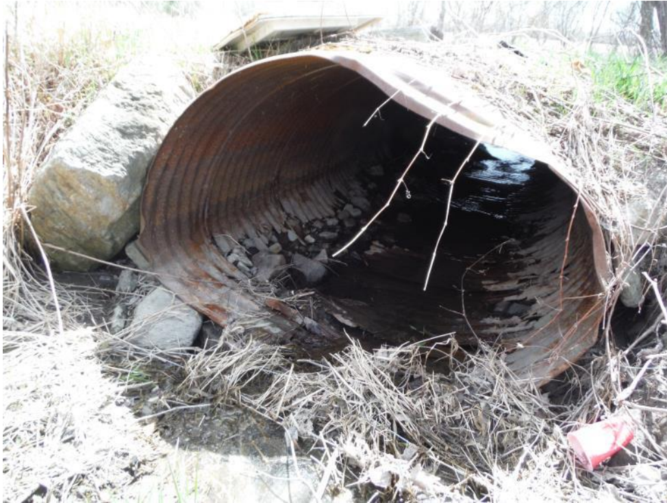
Photo 2 Looking from the upstream end of the culvert to downstream end at the connection to Jock River (May 1, 2015)
