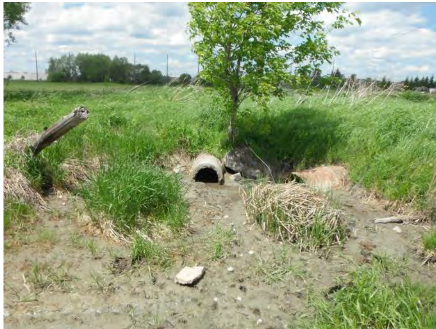
Photo 1 Looking upstream at downstream end of the piped section of the Burnett Municipal Drain (May 21, 2015)
