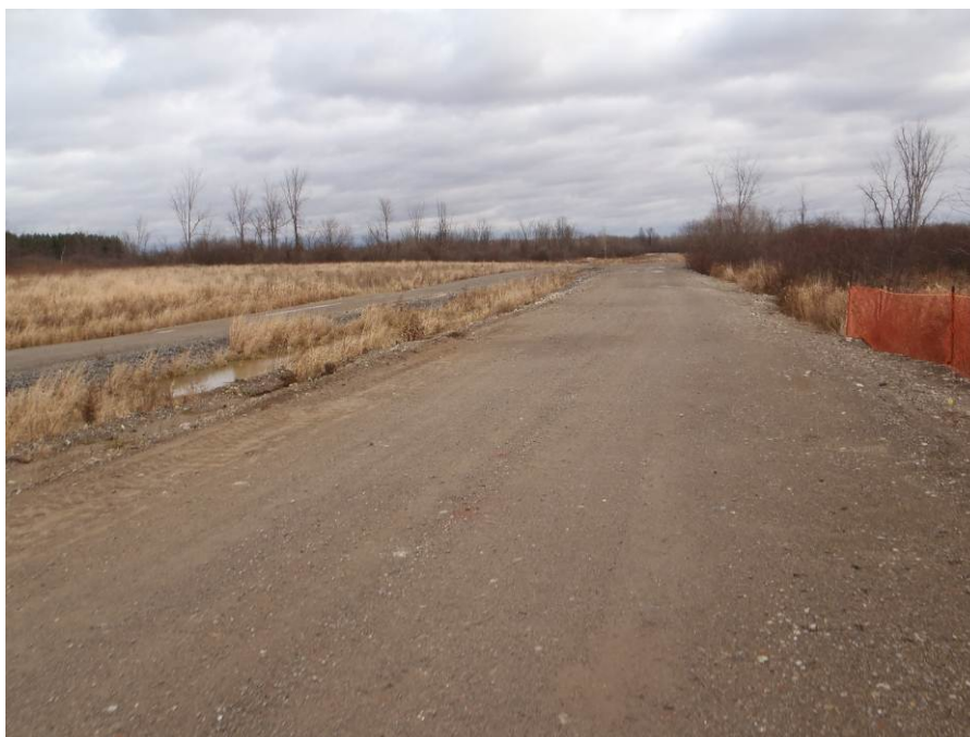
Photograph 2: Looking east towards the access road along the southern Site boundaries.
