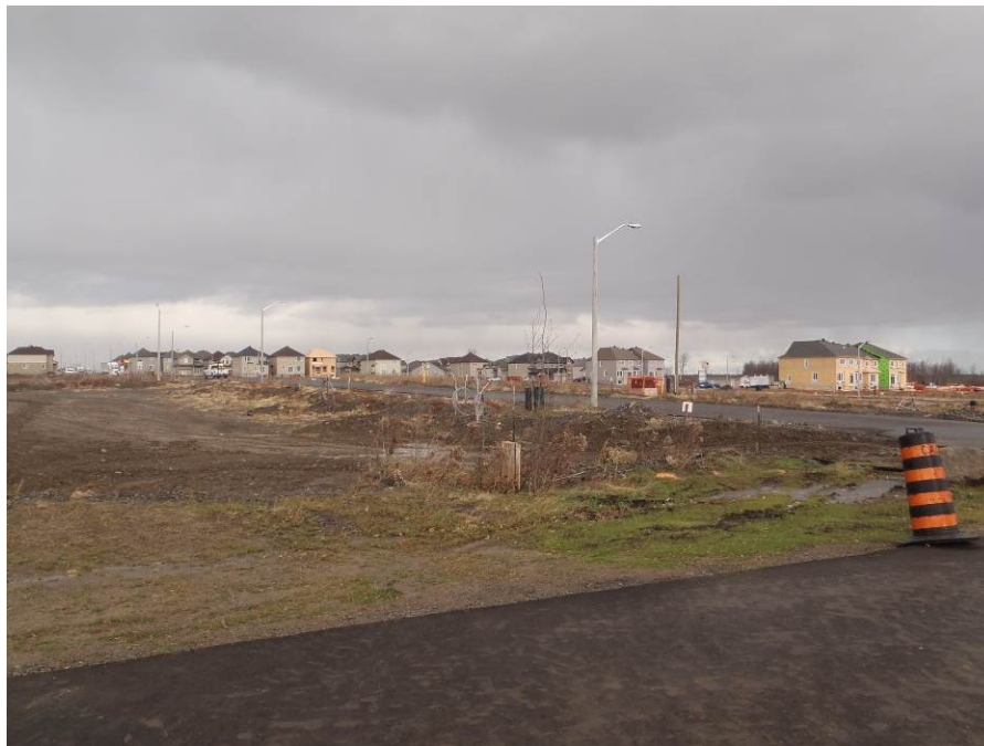
Photograph 19: Looking northeast towards a subdivision that is under construction, located 150 m north of the Site.
