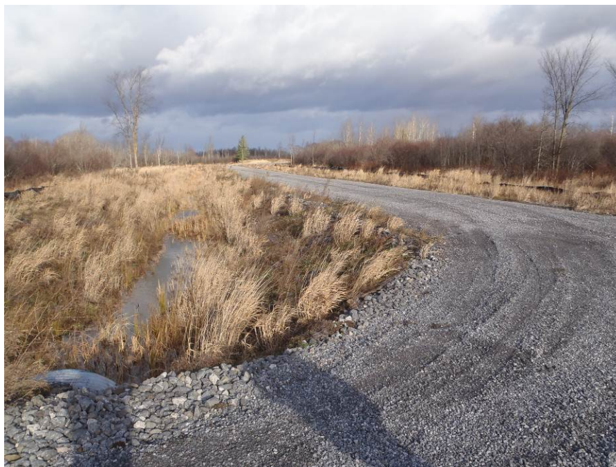
Photograph 6: Looking north towards the intersection where the trunk sanitary and storm sewer alignment splits and runs north-south along the eastern end of the Site.
