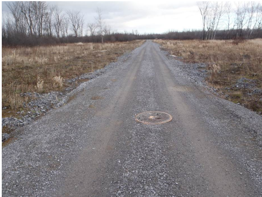
Photograph 4: Looking east along the trunk sanitary and storm sewer alignment with vacant land on the north and south sides of the alignment.
