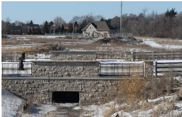
Figure 8: Existing Pumping Station facing north
