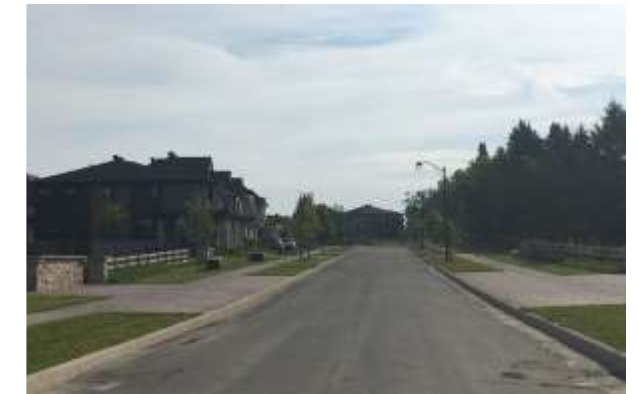
Figure 9: View of Phase 1 from Bridgeport Avenue facing east
