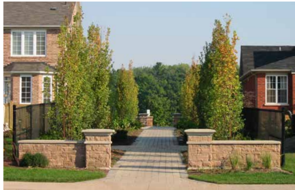
Walkway Block Condition
