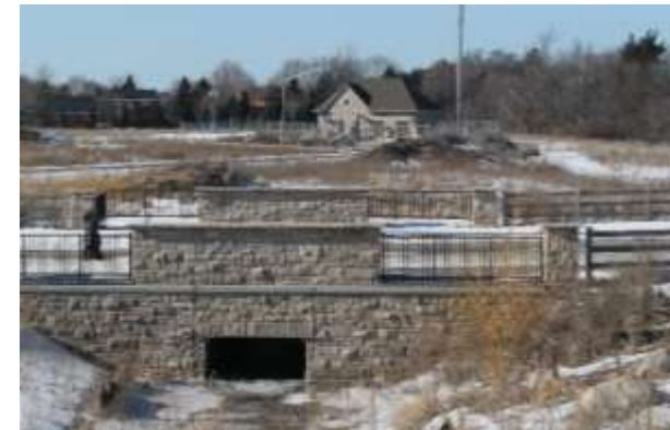
Figure 8: Existing Pumping Station facing north
