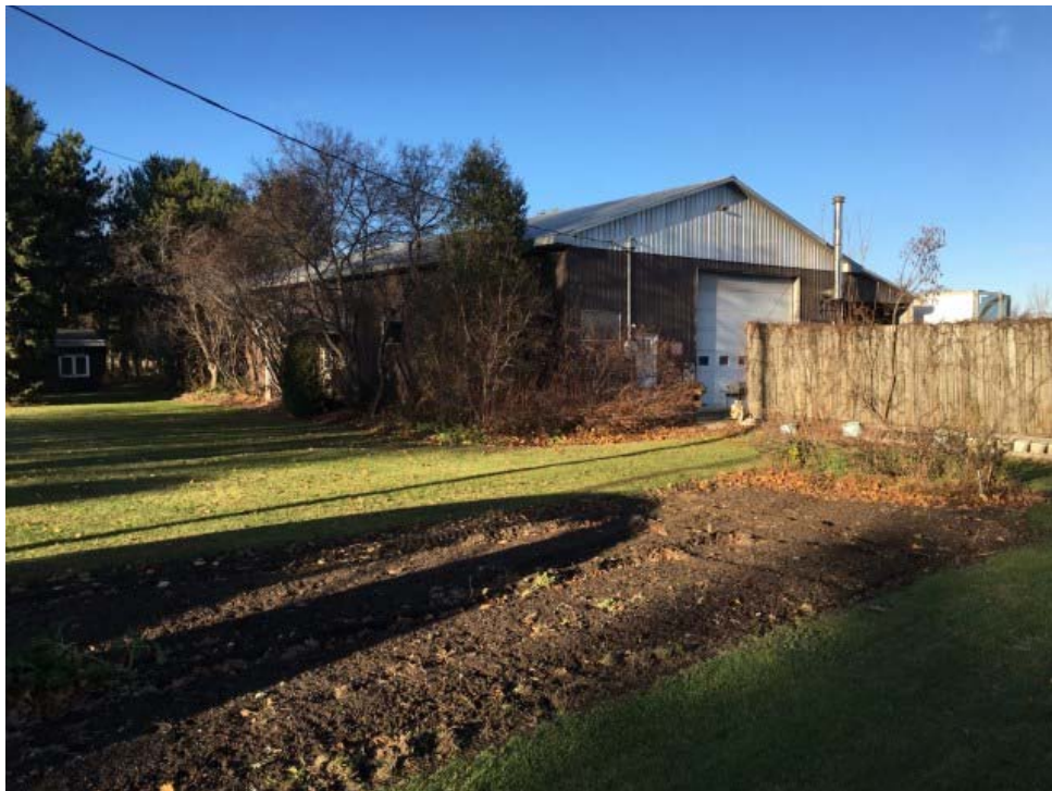
Photo 4: Garage building encroaching the Phase One Property
