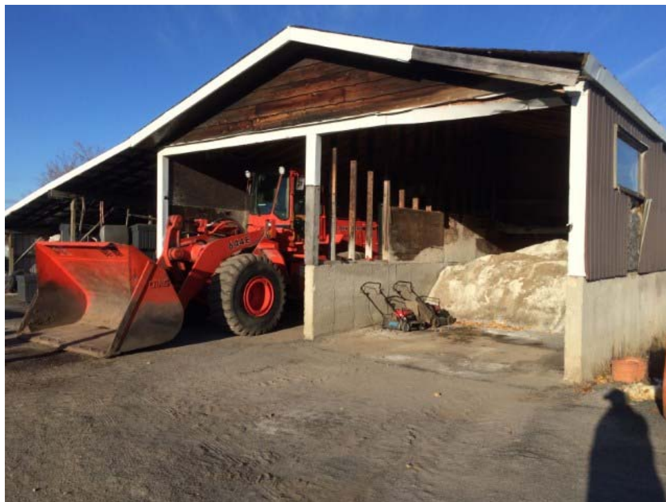
Photo 12: Road maintenance and salt storage building
