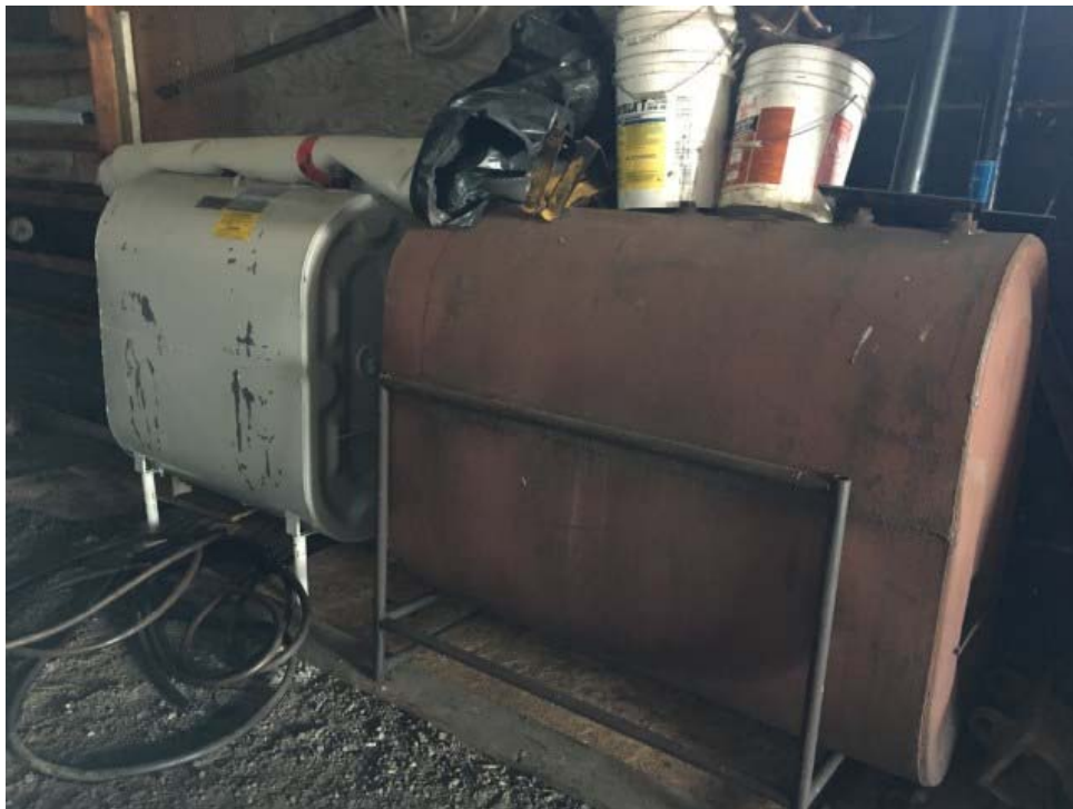
Photo 10: Out of service ASTs
