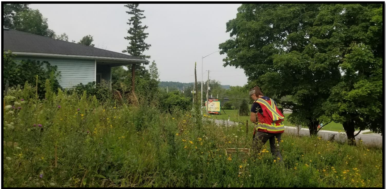
Figure 12: Test pitting around vacant house along Old Montreal Road (D57).
