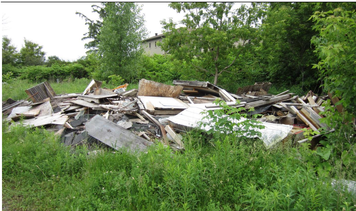
Figure 3. Collapsed farm building, spring 2018
