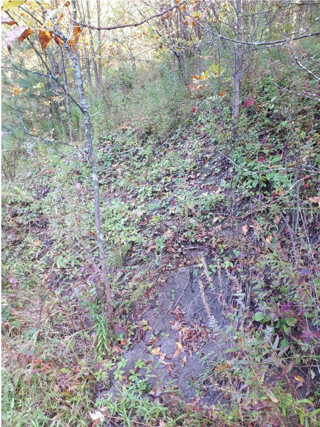
Photograph No. 16: Same sloughing area as Photo 6 viewed from a different angle
