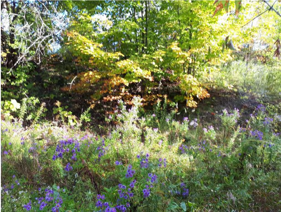
Photograph No. 17: Sloughing of slope, just north of the marsh
