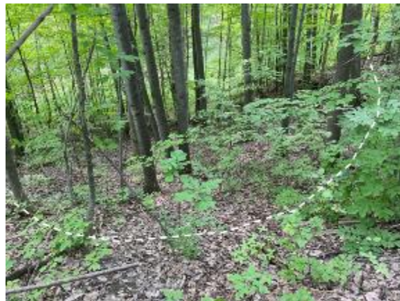
Photo 2: Downslope view of landslide ID 11. Approximate landslide limit in white.
