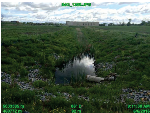
Photo 5 – Reach 2 at culvert discharge/origin of water looking downstream
