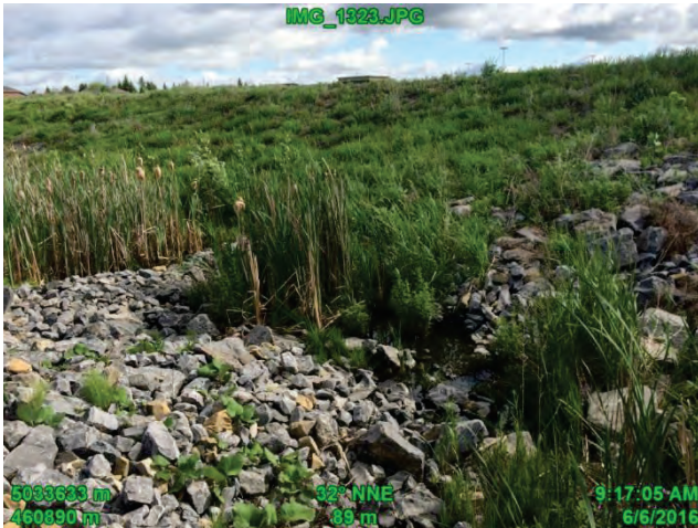
Photo 7 – Typical instream conditions at the 90° bend of Reach 2 – note water is flowing through rip-rap looking downstream
