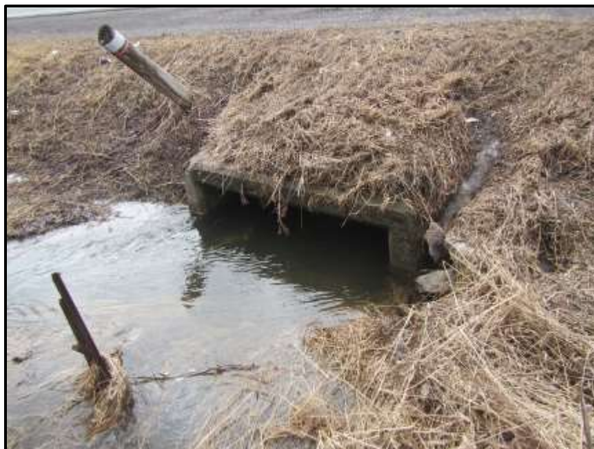
Photograph 3: Survey Site #1 - 2 m concrete box culvert under March Road (facing upstream) (March 30 th , 2018).
