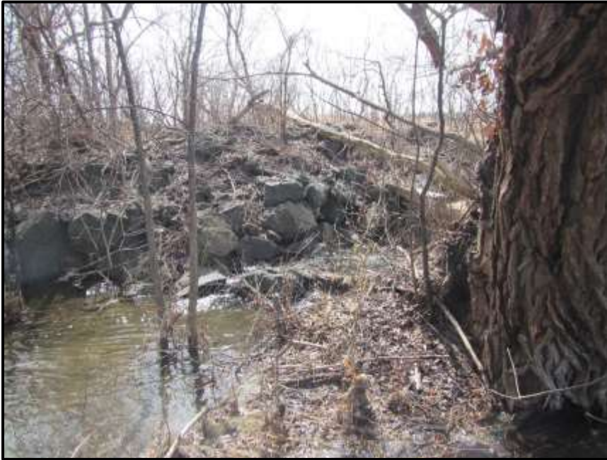
Photograph 7: Old Stone Weir downstream of pond in Survey Site #2 (March 30 th , 2018).
