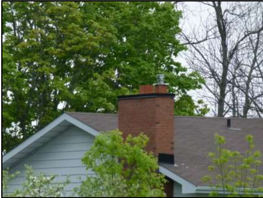
Photograph 35: Chimney at 1145 March Road. Note the ceramic liner and metal cap (May 24 th , 2017).
