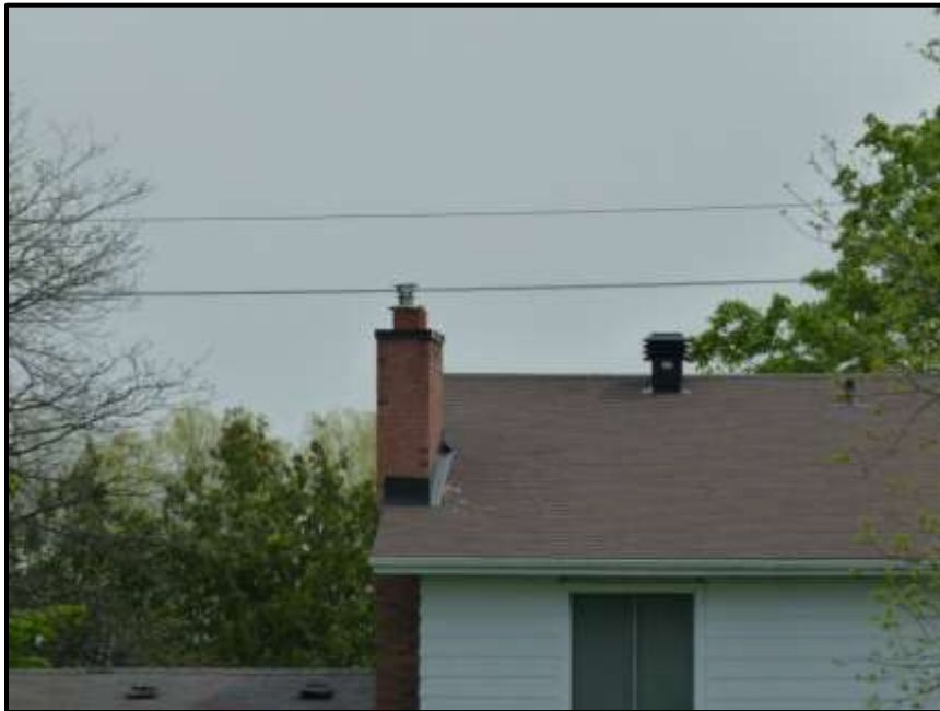
Photograph 33: Chimney at 1053 March Road. Note the ceramic liner and metal cap (May 24 th , 2017).
