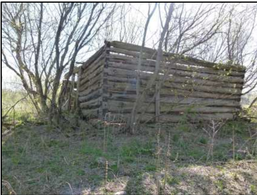
Photograph 46: Building #5 – Looking south at the old barn foundation (May 8 th , 2018).
