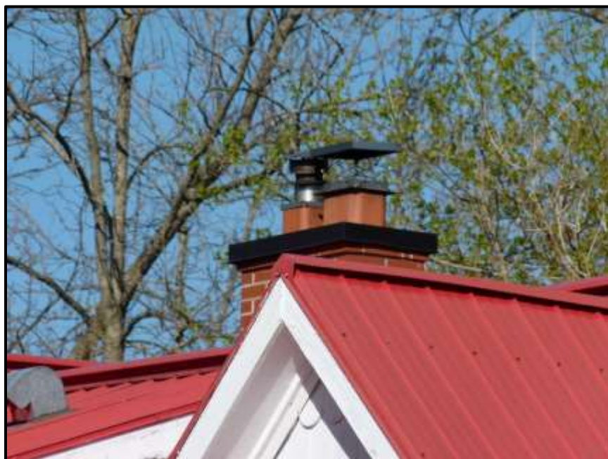
Photograph 42: The capped chimney on the farmhouse at 936 March Road (May 8 th , 2018).
