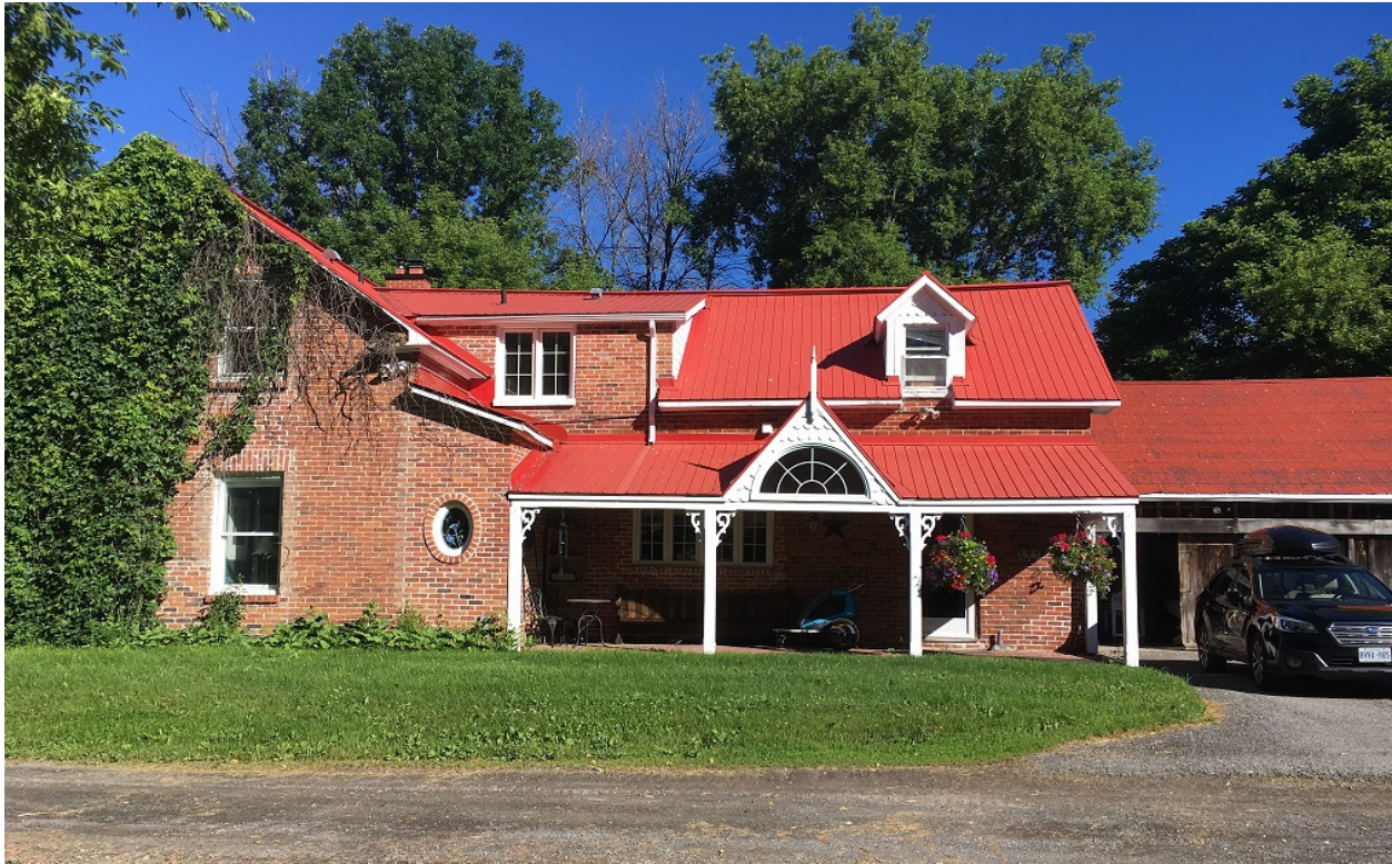
Photograph 1: Photograph illustrates residential dwelling and private garage, facing north.
