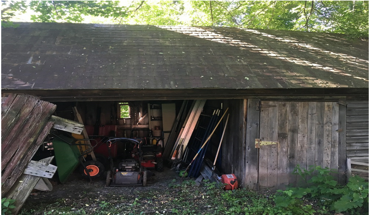
Photograph 3: Photograph illustrates former farm building east of residential dwelling, facing east.
