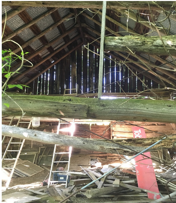
Photograph 4: Photograph illustrates former farm building southeast of residential dwelling, facing west.
