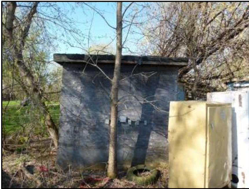
Photograph 44: Building #2 – Looking west at the small wooden shed (May 8 th , 2018).
