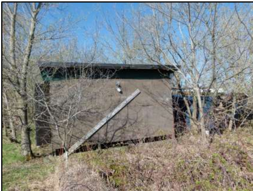
Photograph 45: Building #3 – Looking west at the medium wooden shed (May 8 th , 2018).
