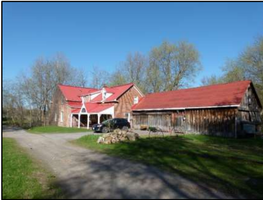
Photograph 42: Building #1 – Looking northwest at the farmhouse at 936 March Road (May 8 th , 2018).
