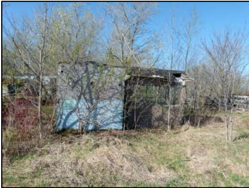
Photograph 46: Building #4 – Looking west at the small wooden shed and glass gazebo (May 8 th , 2018).
