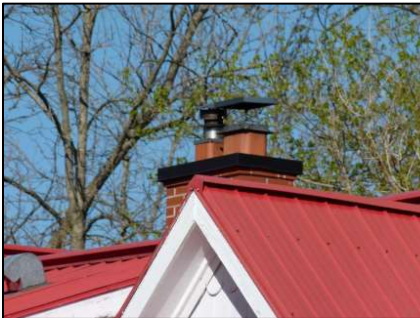
Photograph 43: The capped chimney on the farmhouse at 936 March Road (May 8 th , 2018).
