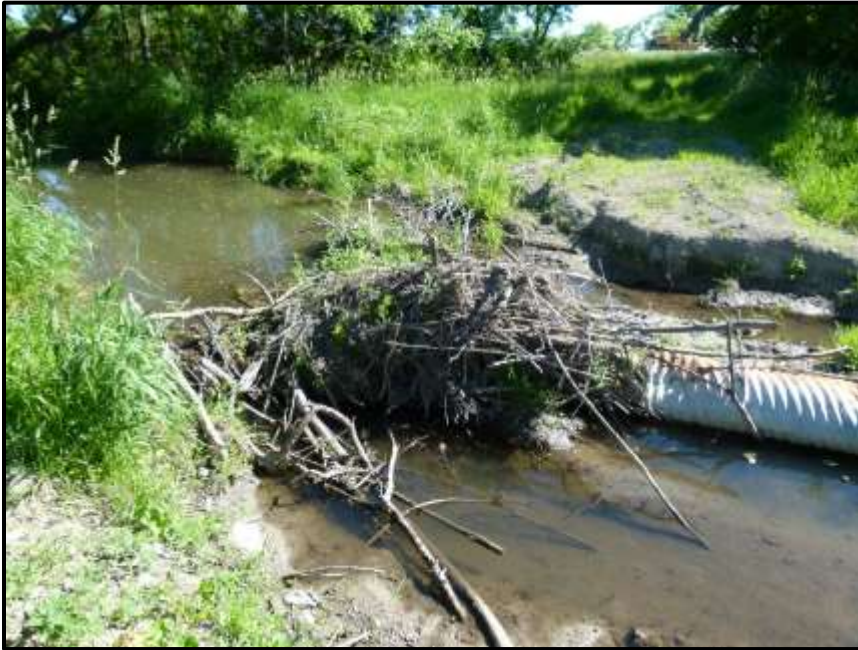
Photograph 37: Looking east at the 900 mm CSP culvert that was historically installed to control water levels associated with a beaver dam. The 900 mm CSP culvert will be removed as part of the habitat enhancement works described in Section 4.2.2 (June 21 st , 2018).
