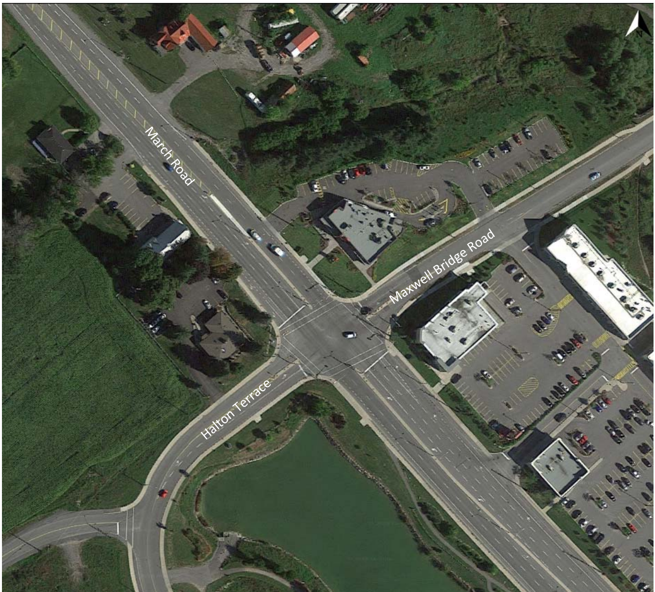
Figure 3: Intersection of Maxwell Bridge Road/Halton Terrace at March Road
