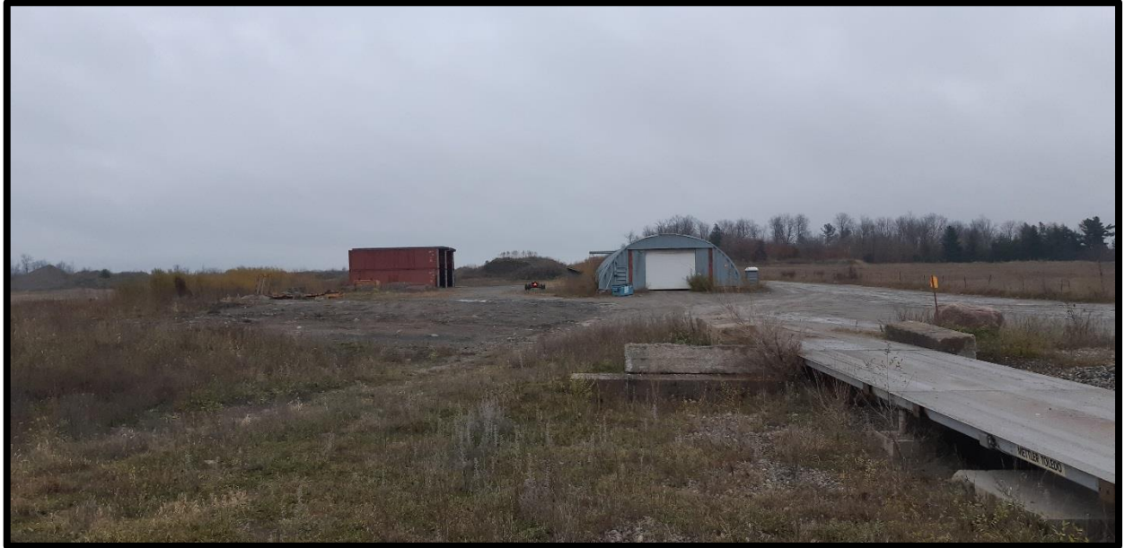
Figure 5: Derelict buildings in southwestern part of the study area. (D016)
