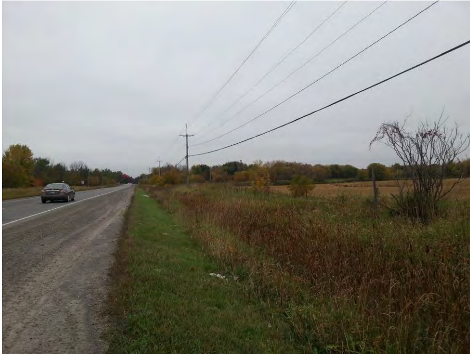
Photograph 1: Looking south down River Road on the eastern edge of Parcel 2. A ditch with cattails lies between River Road and Parcel 2.
