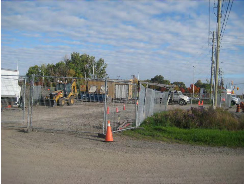
Photograph 3: Looking north from the north-east corner of the Site; trucks and equipment on former construction area for Armstrong-Strandherd Bridge.
