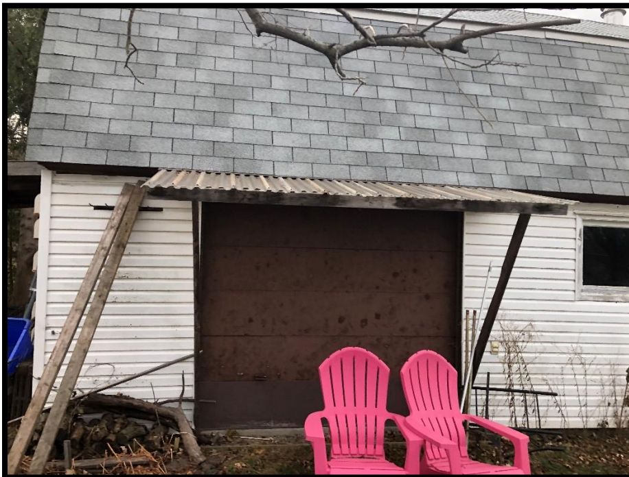
Photograph 6: Northern façade of two storey wood framed workshop, facing south.
