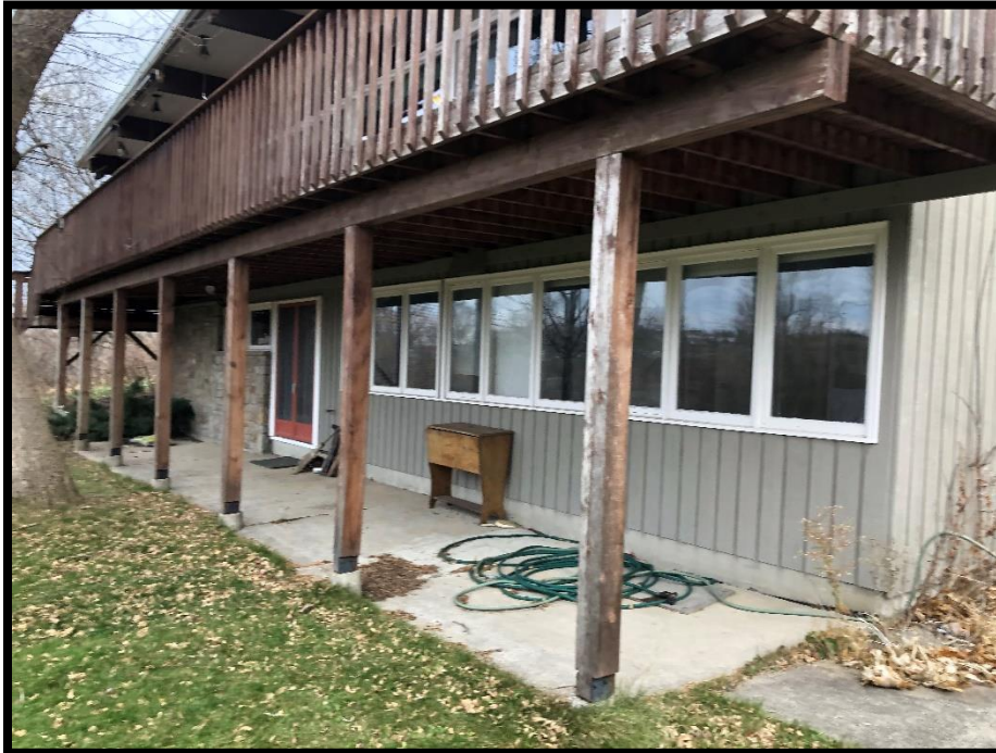
Photograph 3: Rear basement entrance and façade of residential dwelling, facing northeast.
