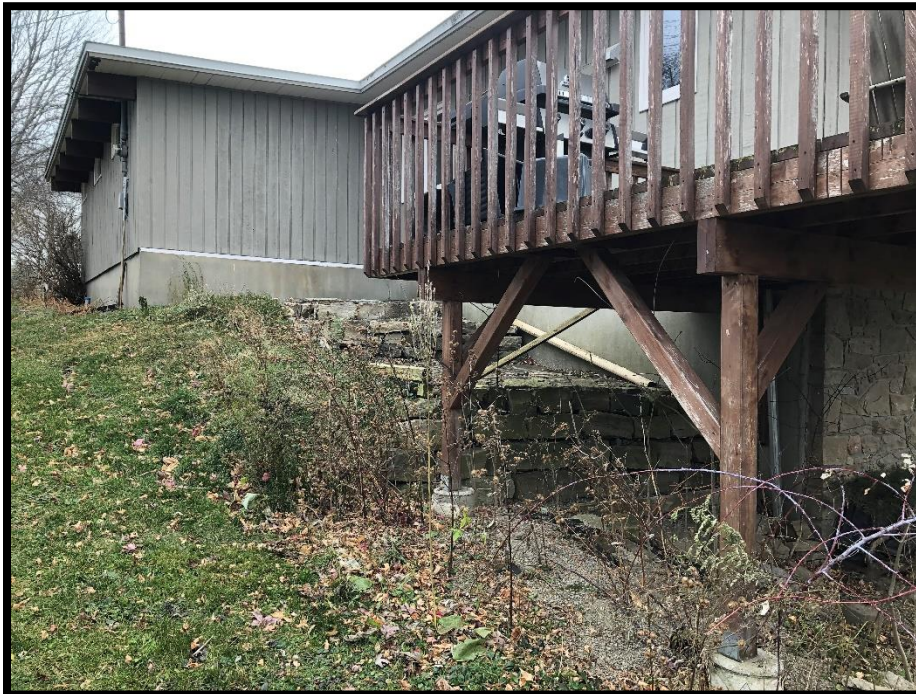
Photograph 4: Northern façade of residential dwelling, facing east.
