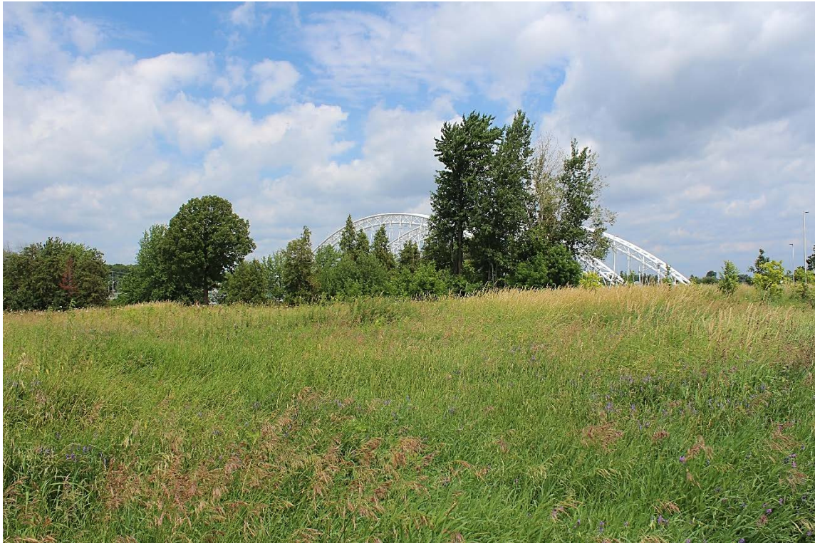
Figure 18: View north from 708 River Road of Vimy Memorial Bridge.
