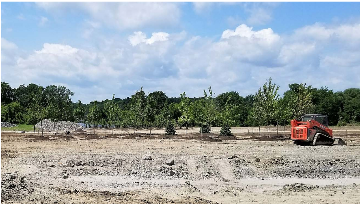
Figure 24: View west of planted trees on 750 River Road.
