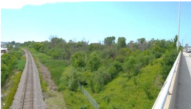
Figure 2-4: Site Looking Northwest on St. Laurent Boulevard (July 17, 2019)
