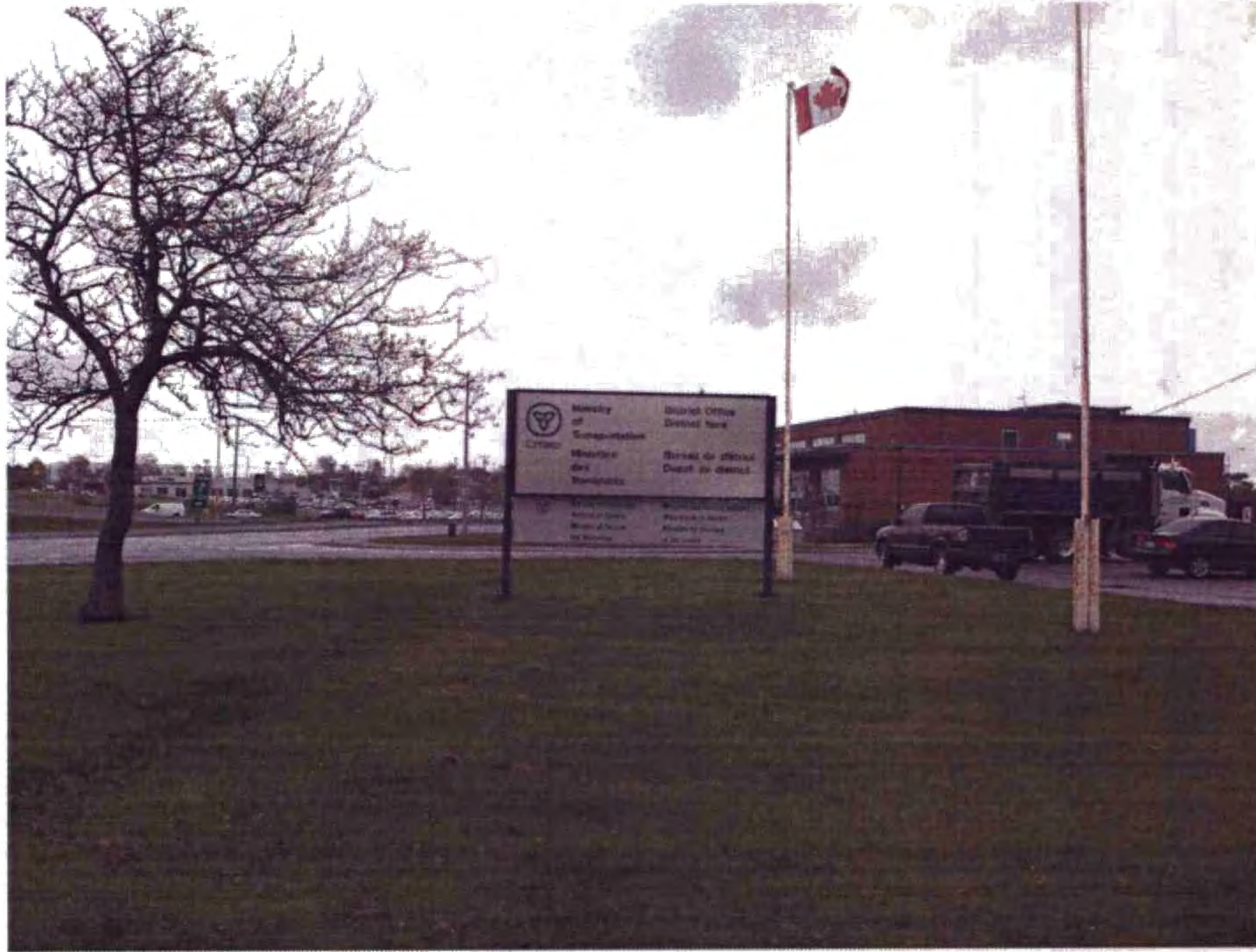
Figure 3: MTO Facility Fronting Tremblay Road, looking east
