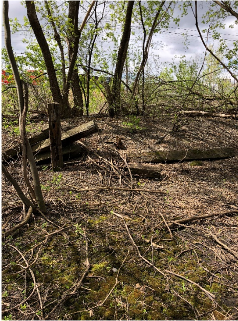
9. Photo of rail ties encountered along the very southern property limit, looking south.
