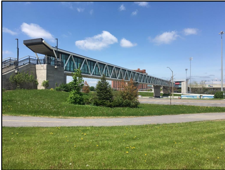
Figure 9: Max Keeping Pedestrian Structure Example
