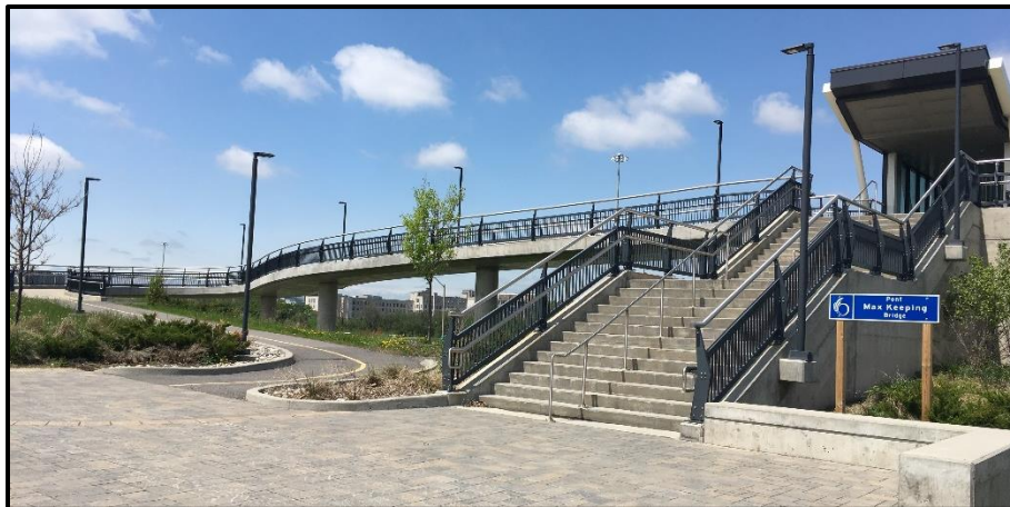
Figure 11: Example of Ramp and Stairs (shown at the Max Keeping Pedestrian Bridge)
