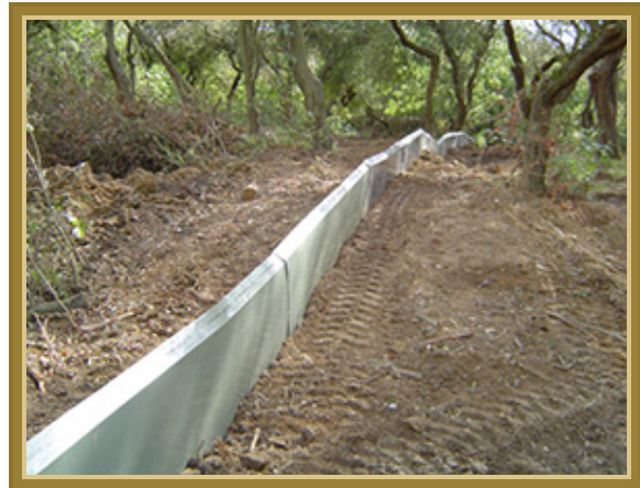
Plate 7. Pre-formed vinyl sheeting fence intended to exclude salamanders for a construction site (photo credit: Herpetosure Ltd.)
