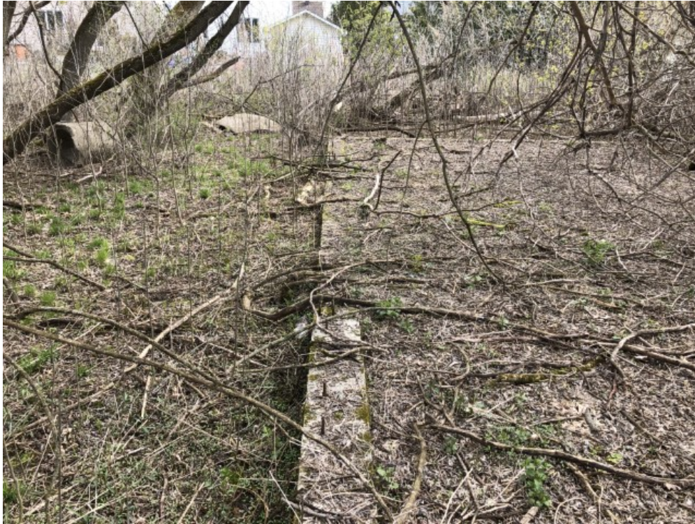
Photo 7: Concrete foundation and concrete debris on the eastern portion of the treed area.
