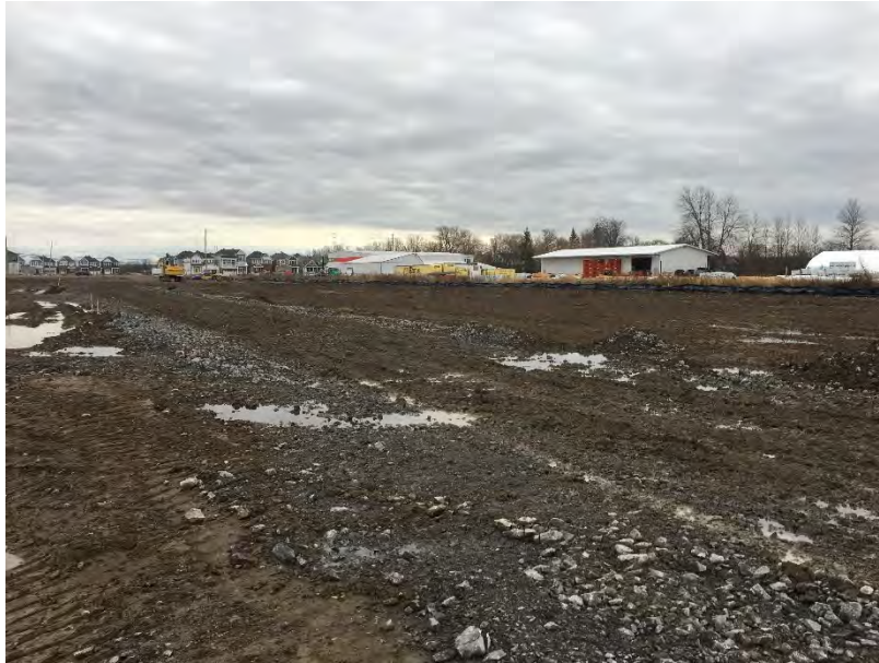
Photo 7 – Looking south at the southern portion of 6363 Perth Street that had been stripped and the adjacent Home Depot property to the west of this property.
