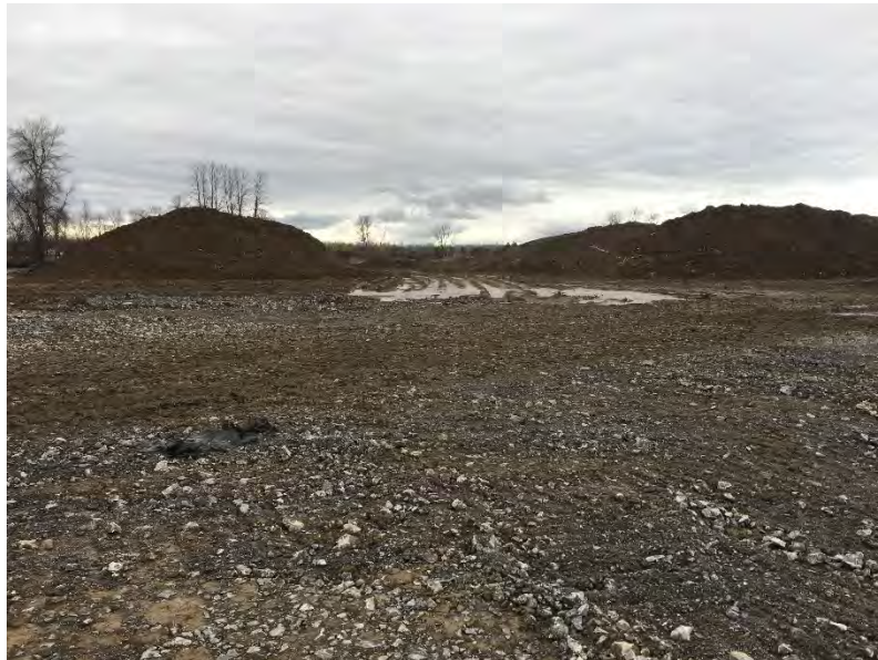
Photo 6 – Looking northwest at the fill piles on the 6363 Perth Street portion of the Site.
