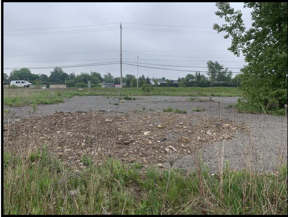
Figure 9: Granular parking area in southwest corner excluded from assessment (PA1183-19E).
