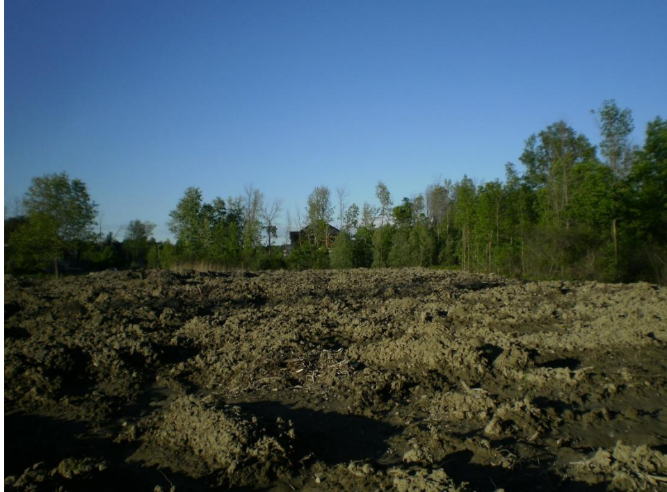
Photo 3 - Fill also dominates the south half of the site. View looking east, with Phase 2 houses in the background
