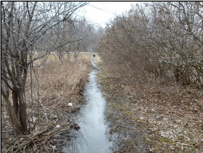
Photograph 10: Looking upstream at the downstream segment of Survey Site #5 (April 4 th , 2022).
