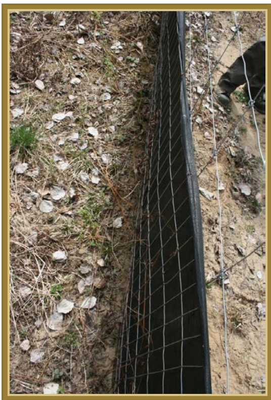
Plate 2. Example of a heavy-duty geotextile fencing used to exclude snake species (photo credit: Jeremy Rouse).
