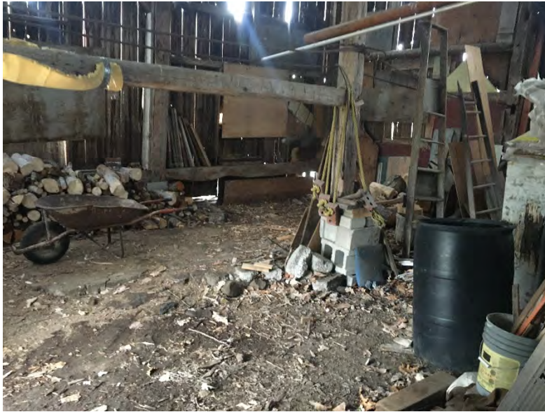
Photo 5 – Photo of the empty drums, wood and storage in the barn.
