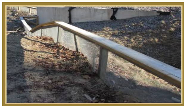
Plate 4. Long-term to permanent exclusion fencing using galvanized mesh with over-hanging lip to prevent animals from climbing or jumping over (photo credit: Megan Bonenfant).
