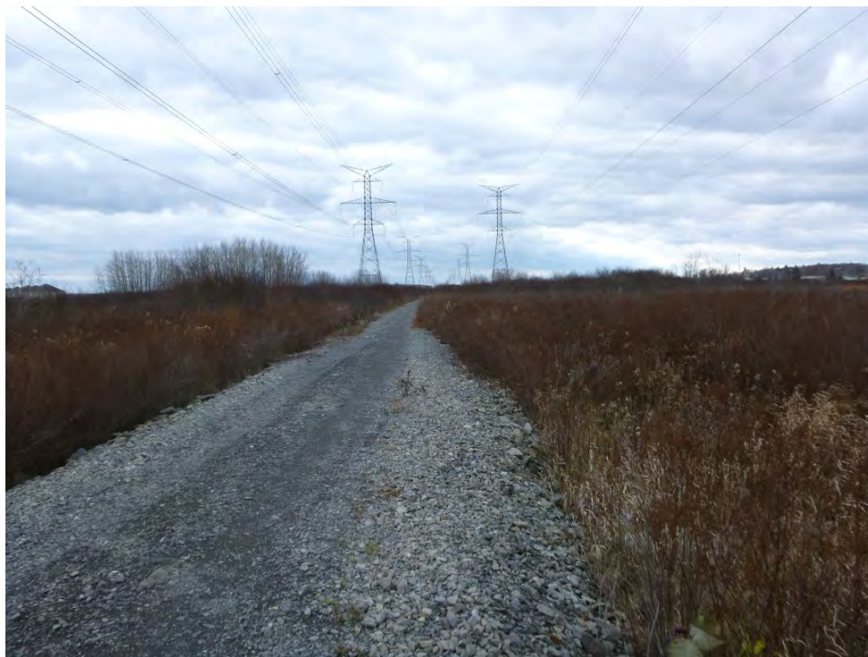
Image 12: Hydro Transmission Line which runs diagonal across the entire study area, looking southwest.
