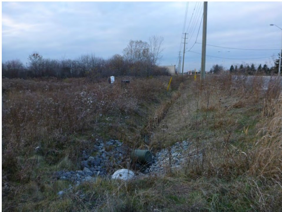
Image 14: Deep drainage ditch disturbance west along Mer Bleue Road, facing northwest.
