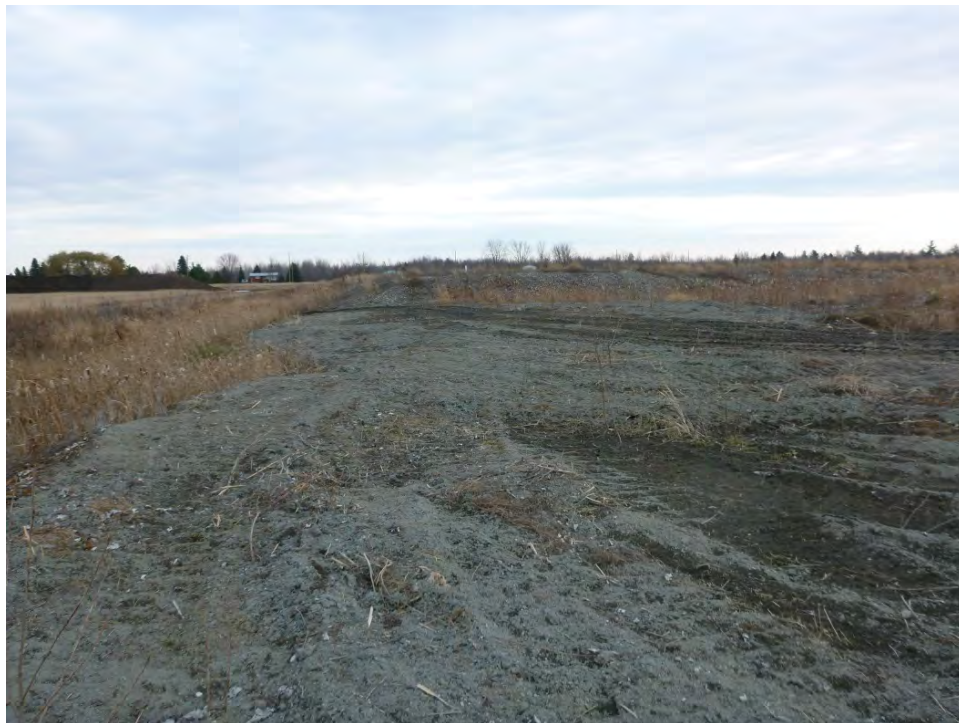
Image 18: Standing above large fill deposit consisting of soil and gravel located along the southern border of the property, looking south.
