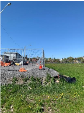
Photo 5: Site conditions on 933 Gladstone Av. Facing west
