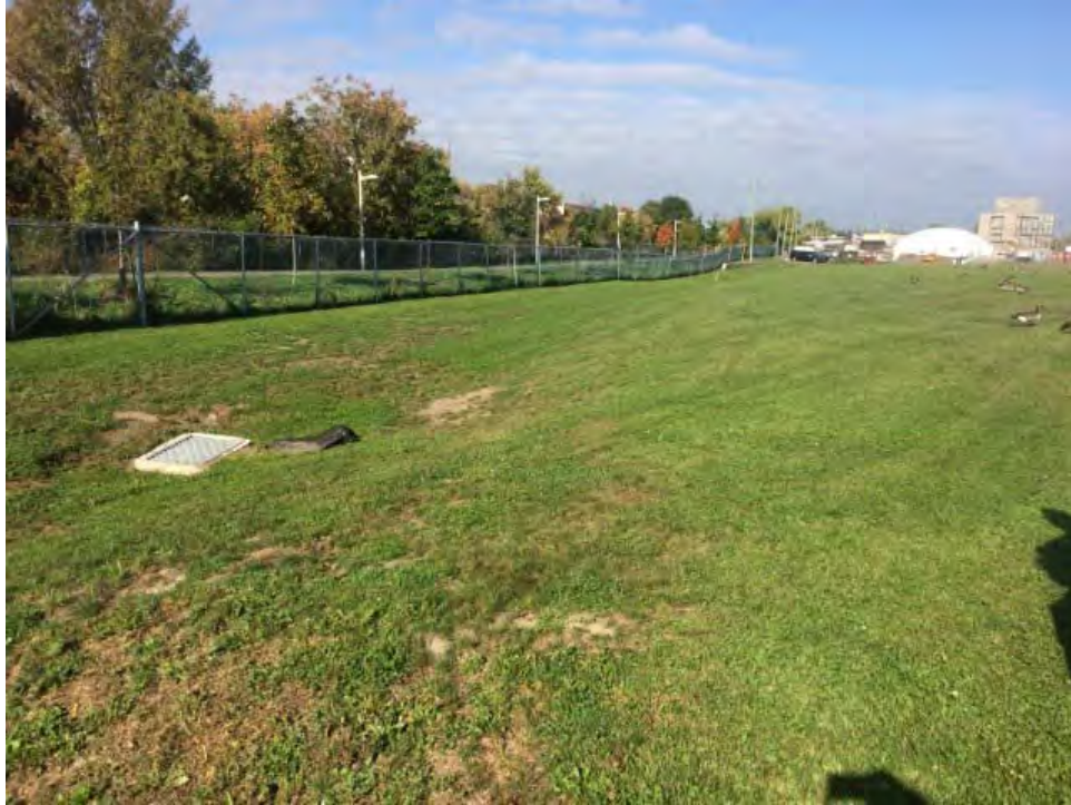
Photo 7: Storm drain, 933 Gladstone, Facing northwest from southern edge of Site beside Gladstone Ave.
