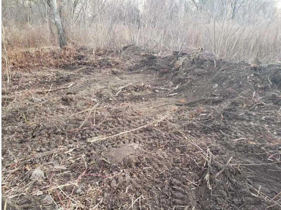
Photographs of surface of test pits 3 and 4, Nov. 8, 2022 after asphalt debris removed from test pits
