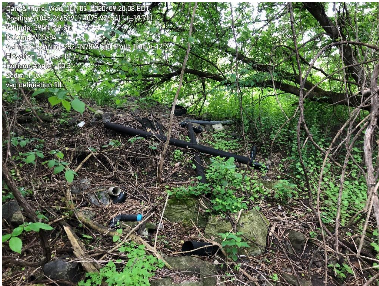
Figure 10 Photo of fill and rubble on the edge of the wetland on the Site
