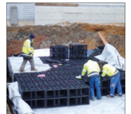
Industrial building, Tumeltsham (AT)
