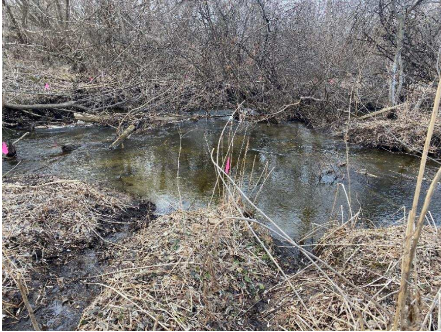
Gully erosion at the Poole Creek west of cross-section A
