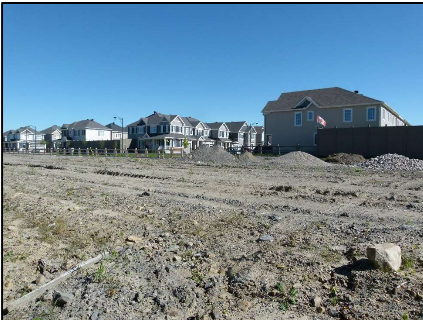
Photograph 11: Looking south at the adjacent residential subdivision. The area shown historically included the upstream portion of Drainage Feature A (September 17 th , 2020).
