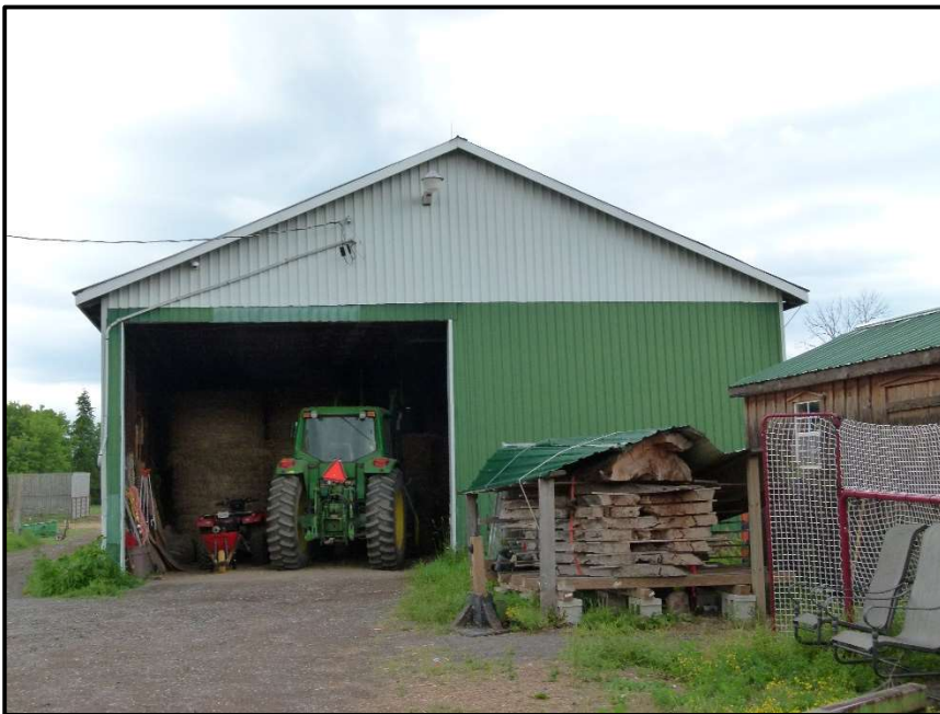
Photograph 18: Structure #2 (Tractor Garage). Two (2) active Barn Swallow nests were observed within Structure #2 (July 29 th , 2020).
