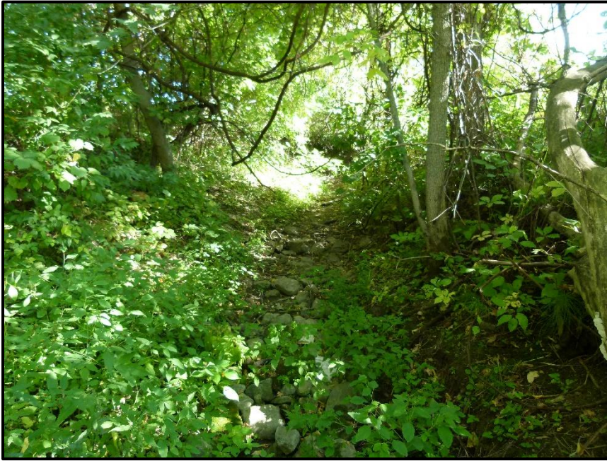
Photograph 14: Looking south at the northern end of the remnant portion of Drainage Feature C (September 17 th , 2020).
