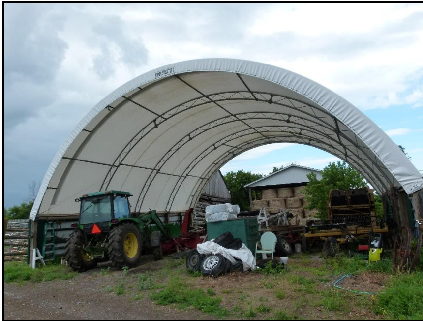
Photograph 21: Structure #3 (Plastic Coverall). No Barn Swallow nests were observed within Structure #3 (July 29 th , 2020).
