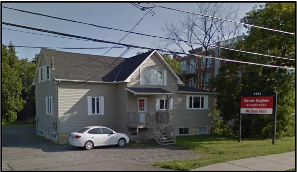
Photograph 6: View of the two-storey commercial/residential building on the northwestern portion of the site. Photograph taken facing southwest.
