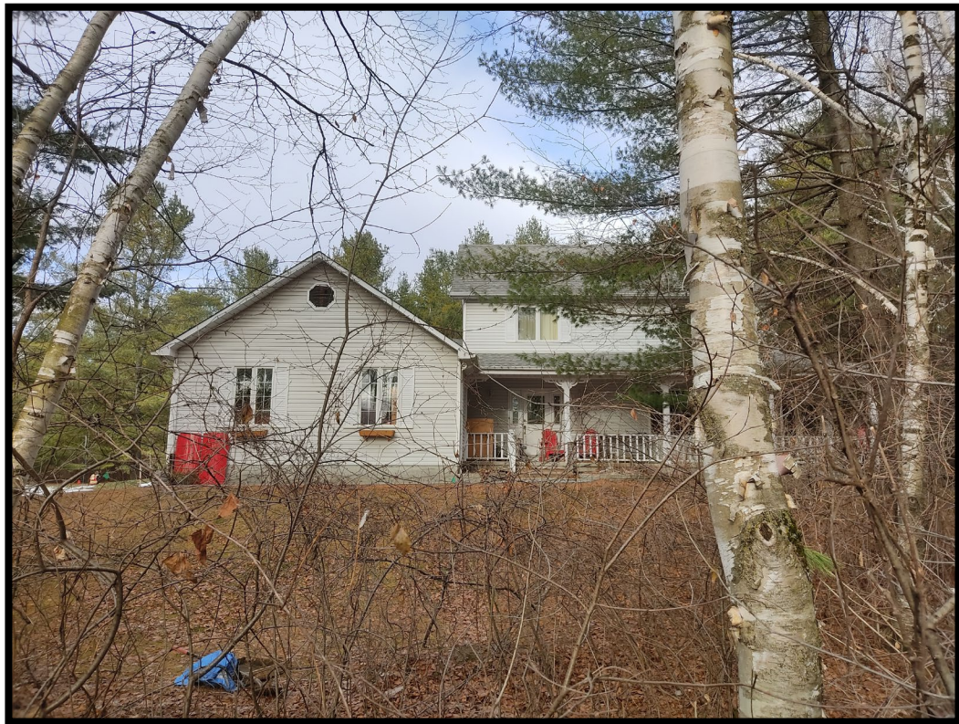
Figure 4: Testing in front of house (PA1215-D45).
