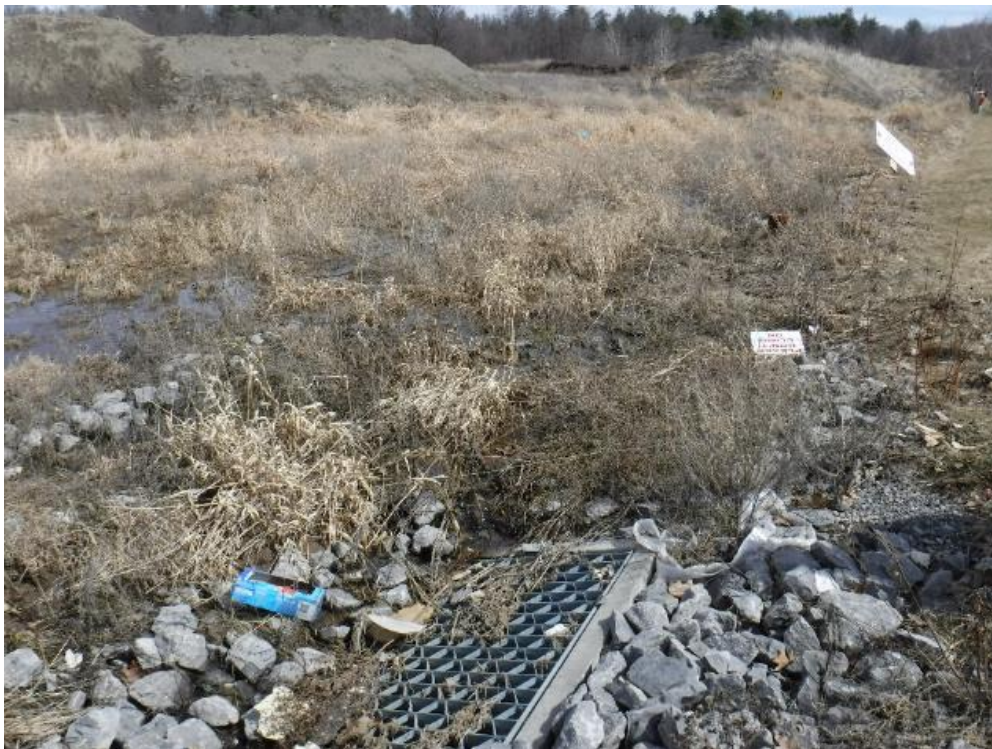
Photo 4: Looking upstream by inlet catch basin (March 30, 2021)
